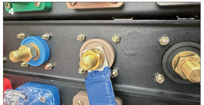
Refit the washer and nut onto the threaded post, then tightn to max. of 12N/m
