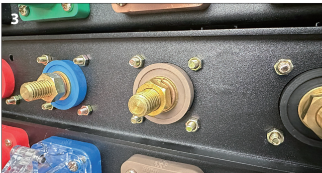
Fit the terminal over the threaded post
